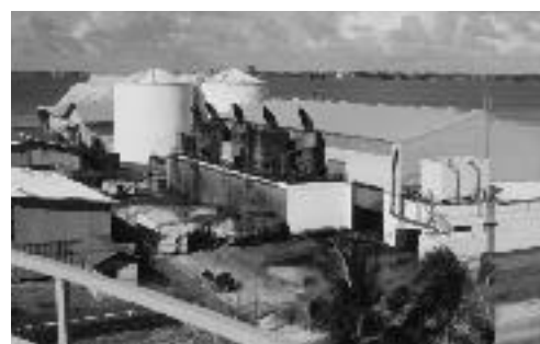
Power plant, Majuro
